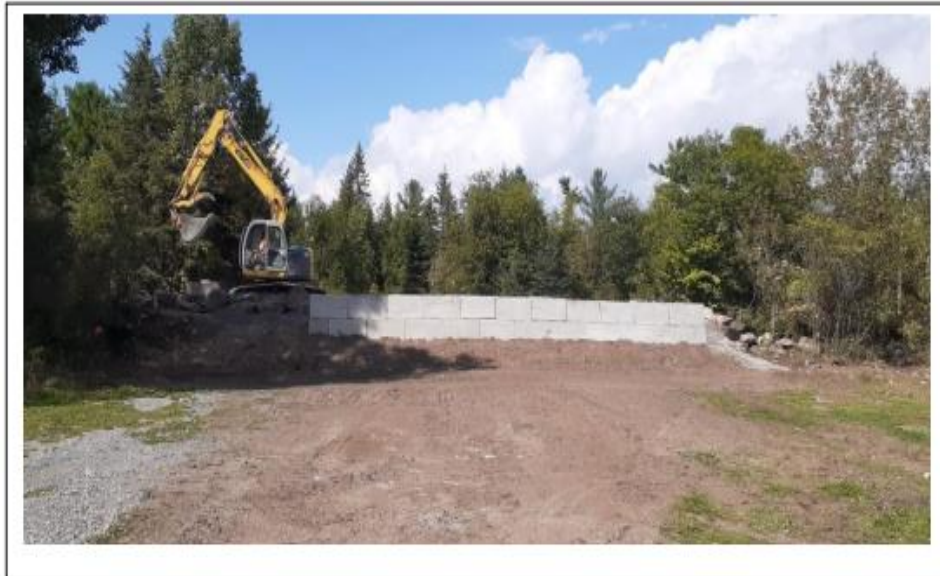
Photo 7: Construction of a large barricade (Phase III) at location of ramp.
