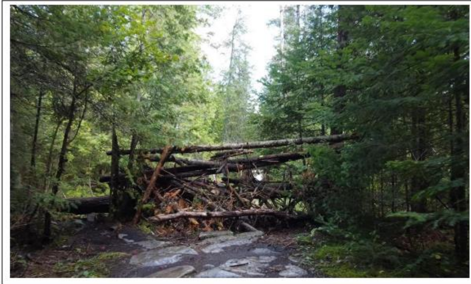
Photo 3: Mucking Trail barricade constructed from local materials and volunteer labour. Note that forest soil was worn away down to bedrock by ATVs.
