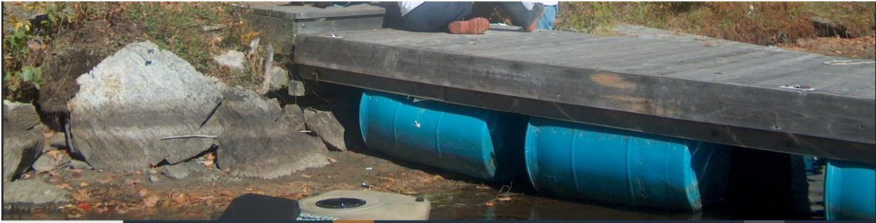
Pictures of existing floating docks at the Ferguson property:
