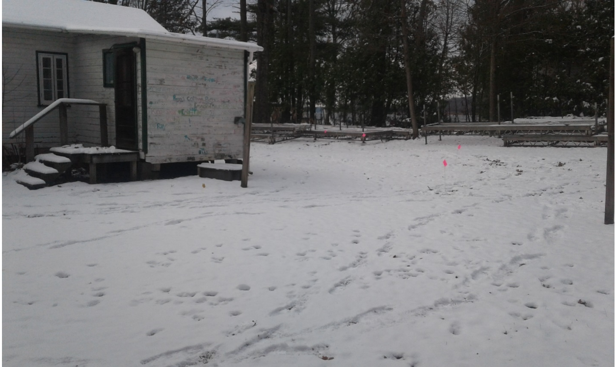
Figure 15: Looking southwest towards the north side of the dwelling. Pink flags demonstrate the approximate flood plain (November 18, 2022).
