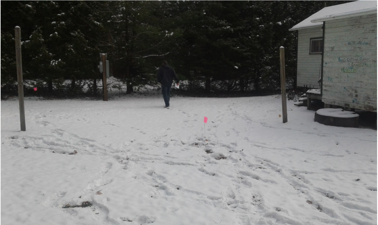
Figure 12: Looking east towards the north side of the dwelling. Pink flags demonstrate the approximate flood plain (November 18, 2022).
